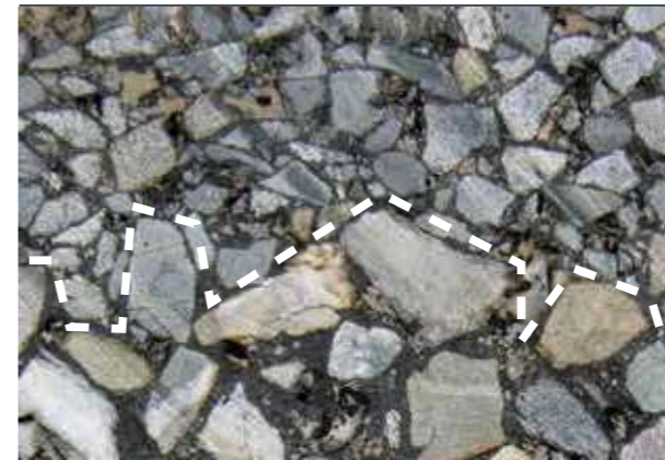
Excellent bond and interlocking of binder and surface courses
