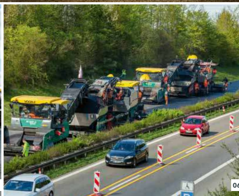
04 Pavement rehabilitation of a motorway at night. 05 Pavement rehabilitation of a rural road: 10 cm binder course and 2 cm surface course were paved in 12-hour shifts – no problem for the InLine Pave train. 06 Rehabilitation of lorry lane. Traffic kept flowing on the adjacent lane.
