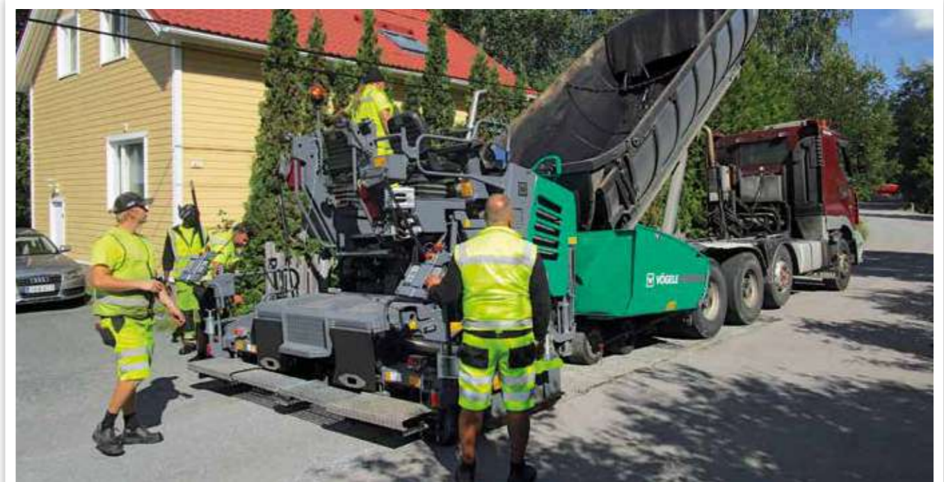
PAVEMENT REHABILITATION ON MUNICIPAL ROADS
