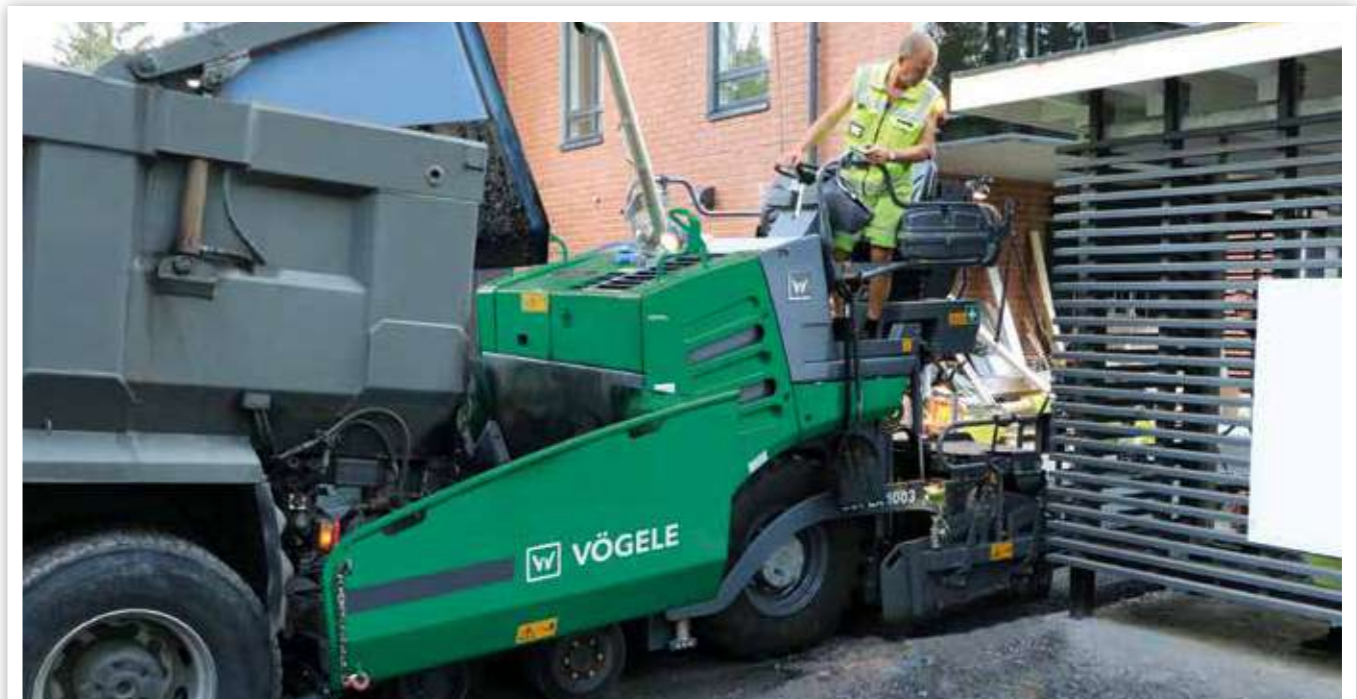
REHABILITATING ACCESS ROADS
